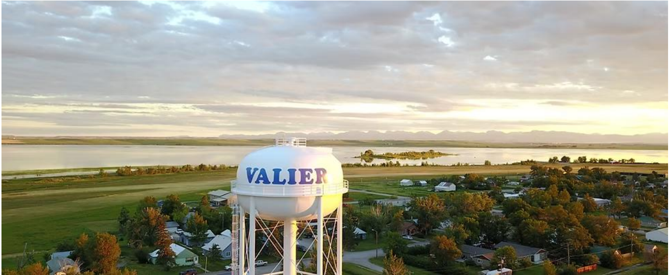
Photo courtesy of Valier Development Corporation
